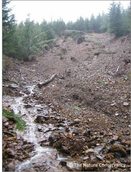
Image 2. Landslide initiated from road
